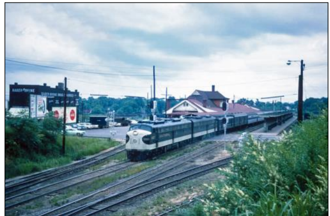
The Crescent prior to being taken over by Amtrak.
