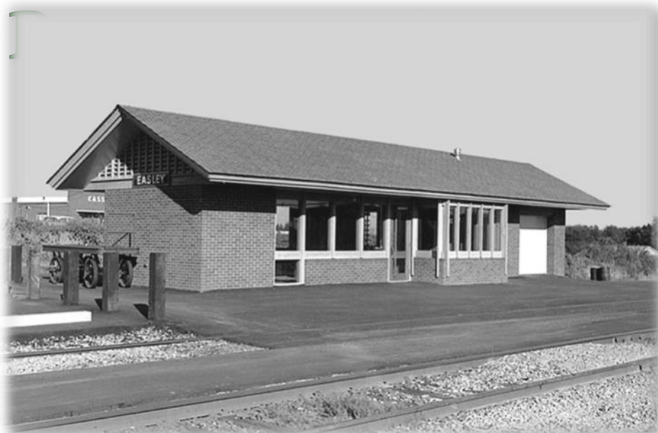
The new Southern Railway Easley depot. Located near the intersection of Dennis and Hagood Streets.
