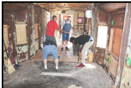
Members remove flooring as work continues on the caboose restoration.
