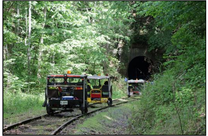
Approaching one of two tunnels on the line.
