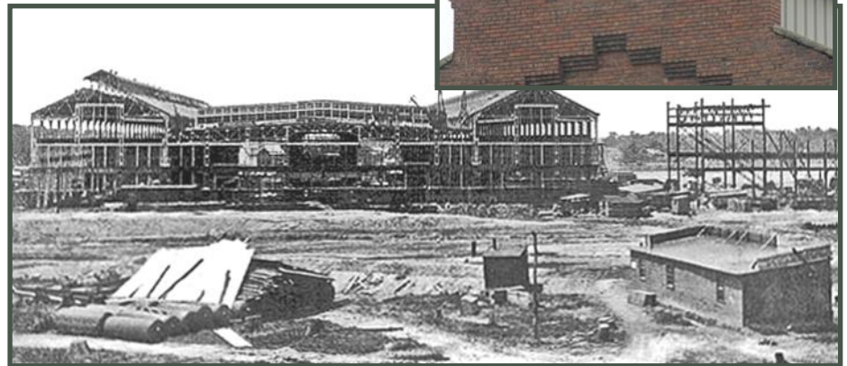
Shop construction circa 1910 and modern day view of parapet.
