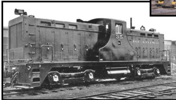
The St. Louis Car Company/Fairbanks-Morse 600-horsepower center-cab switcher #35 was truly a unique locomotive on the Reading, had two 300-horsepower in-line engines for power.
