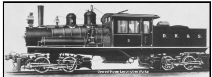
An unusual design Vulkan Duplex built to compete with Shay locomotives.
