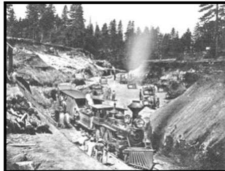
Building the CP in western Utah.
