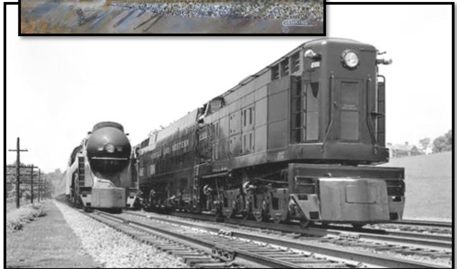
The N&W "Jawn Henry" was a 4500hp brute. It totaled over 111 feet long. Seen with #611 the extreme length is obvious.
