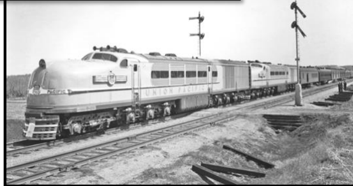
Photo of the Union Pacific GE steam turbine locomotives, April 1939. Photo at right shows the loco with an unusual dark paint scheme.
