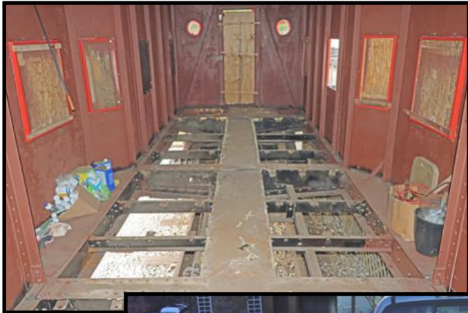
↑ Floor completely removed.
