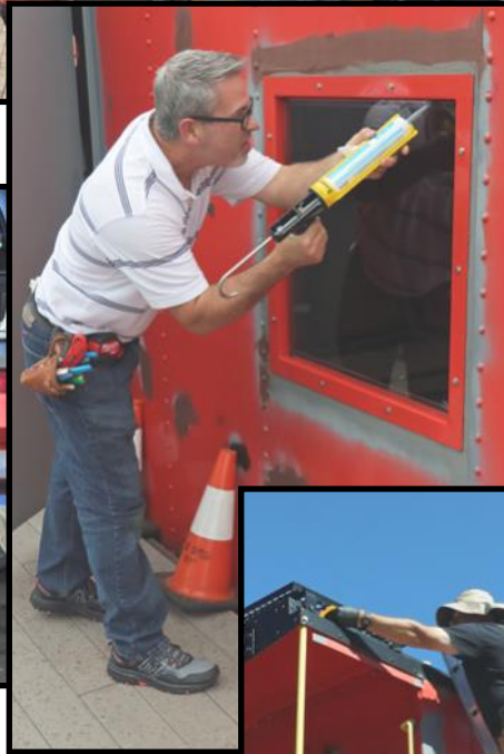
← Sealing up the new glazing.
