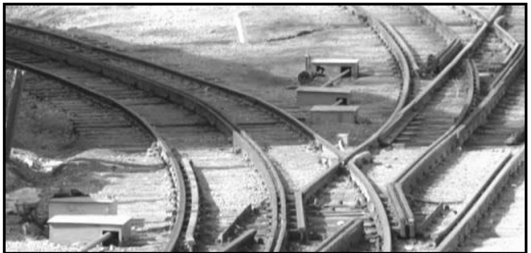
Operation of a cog turnout is not a single step operation, many parts need to be moved.
