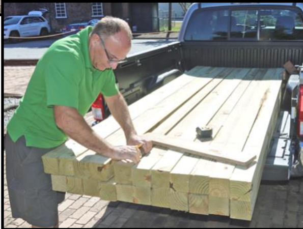
New 4x4 → floor joists.
