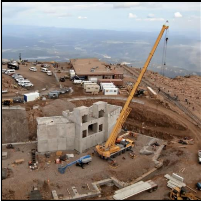
↑ New summit visitor center under construction.
