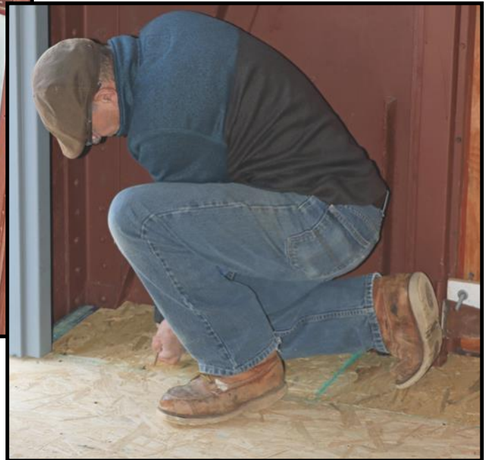
Caboose interior with studs waiting for installation. ↑ Duane putting in the last of several hundred screws in the floor sandwich of plywood, insulation, and OSB. →
