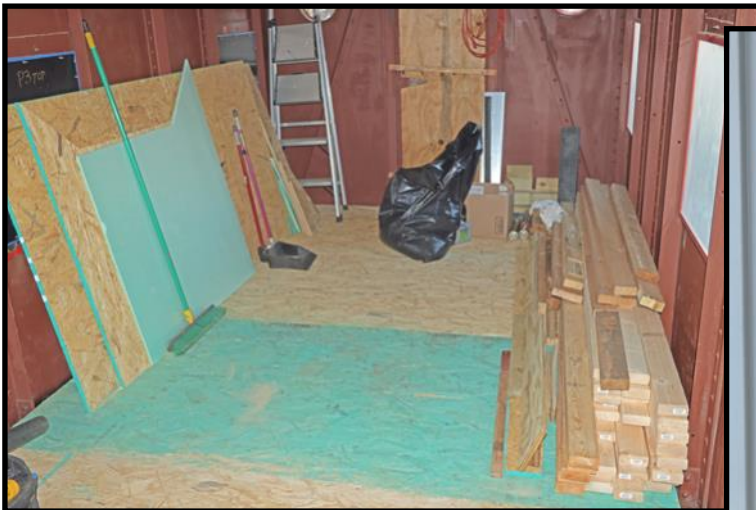
Caboose interior with studs waiting for installation. ↑ Duane putting in the last of several hundred screws in the floor sandwich of plywood, insulation, and OSB. →
