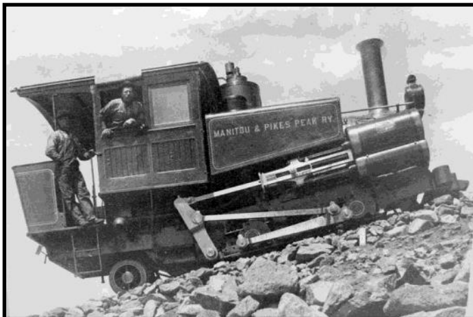
Lever drive used on steam locos.
