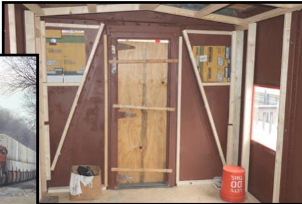
↑ No nails used in construction. White plastic spacer to keep wood away from metal.
