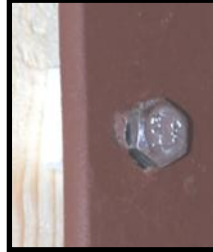
↑ No nails used in construction. White plastic spacer to keep wood away from metal.
