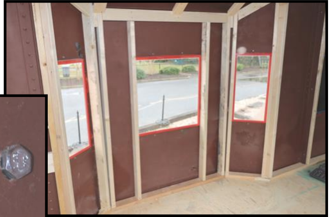
↑ No nails used in construction. White plastic spacer to keep wood away from metal.
