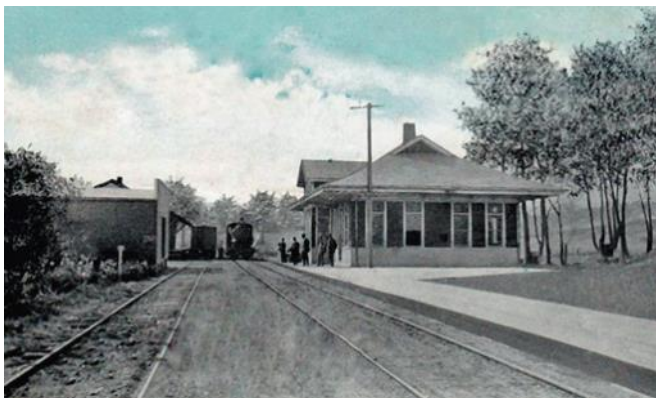
Blue Ridge Railway end of track at Walhalla, SC.
