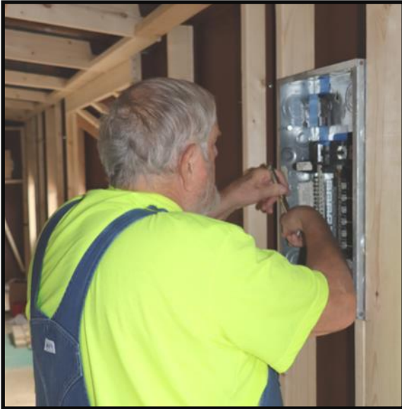
Electrical panel box being installed by Pat O'Shields.
