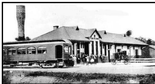
Piedmont & Northern car stopped at Belton, SC station.
