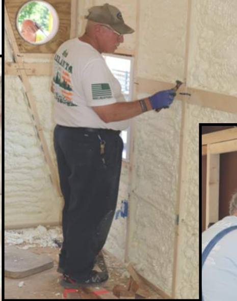
Pat and Bruce → work on wiring the electrical panel. Some of us have been working here too long and need a haircut.
