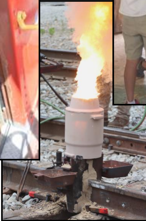
↑ Thermite welding new rail in the Magnolia Street crossing.
