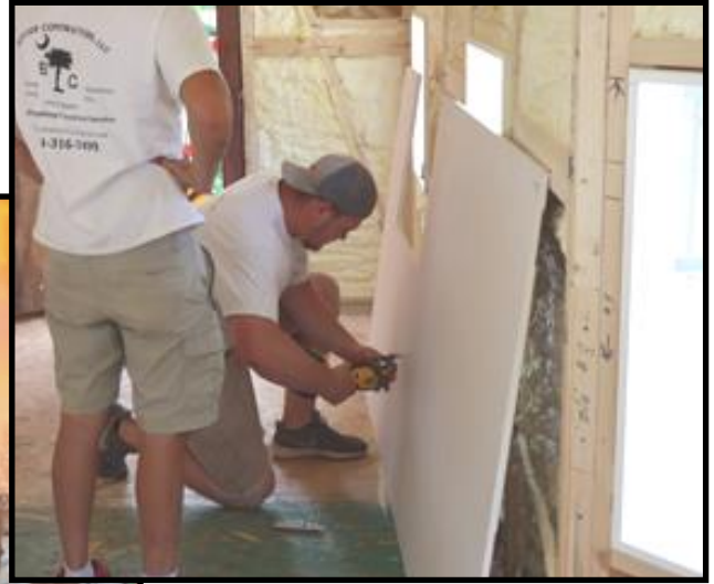
↑ Drywall installation begins in the caboose.
