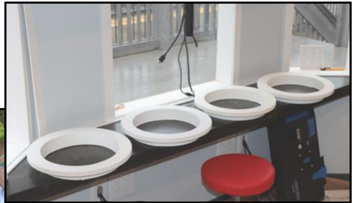
Custom made plastic interior portal window trim ready for installation.
