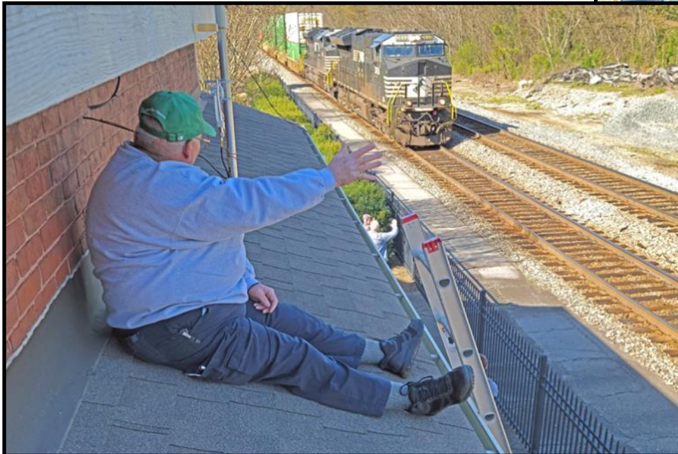
↑ Bob Klempner shown working(?) on the Wi-Fi antenna installation on the depot which afforded him a unique railfan location to watch trains.
