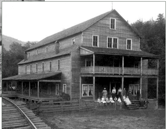
Hotel served by the Clinchfield at Unaka, NC.
