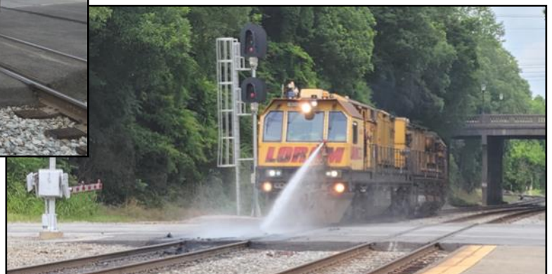
After the rail grinding train passes a following train extinguishes any fires in the ties and washes off the debris from the crossing. →
