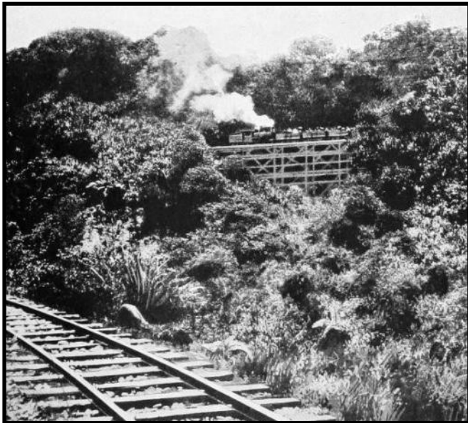
Shay locomotive rounding a horseshoe curve of 164 foot radius 5% upon Mount Arisan Railway, Formosa.
