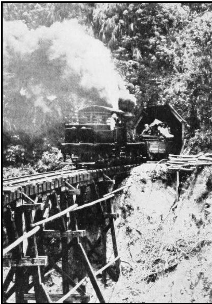
The hill climber Shay ascending a grade of 5% on the Mount Arisan Logging Railway in Formosa.
